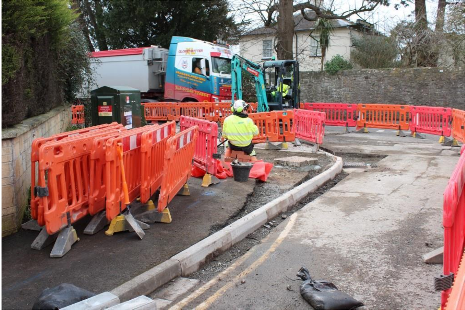
Barberry Farm Road/High Street corner – tightening the road junction radius and widening the pavement
